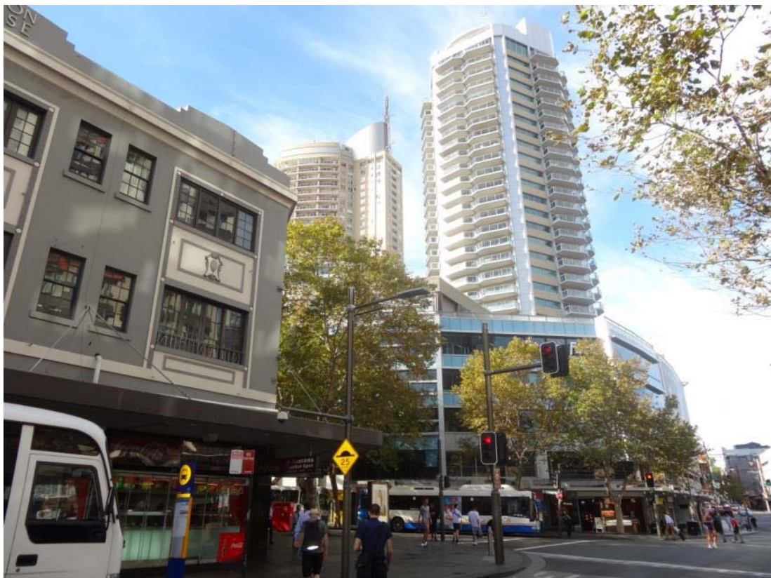
Figure 10: View towards the Zenith building at 82-94 Darlinghurst Road, located to the south east of the site, and a partial view of Minton House (left) directly opposite the subject site
