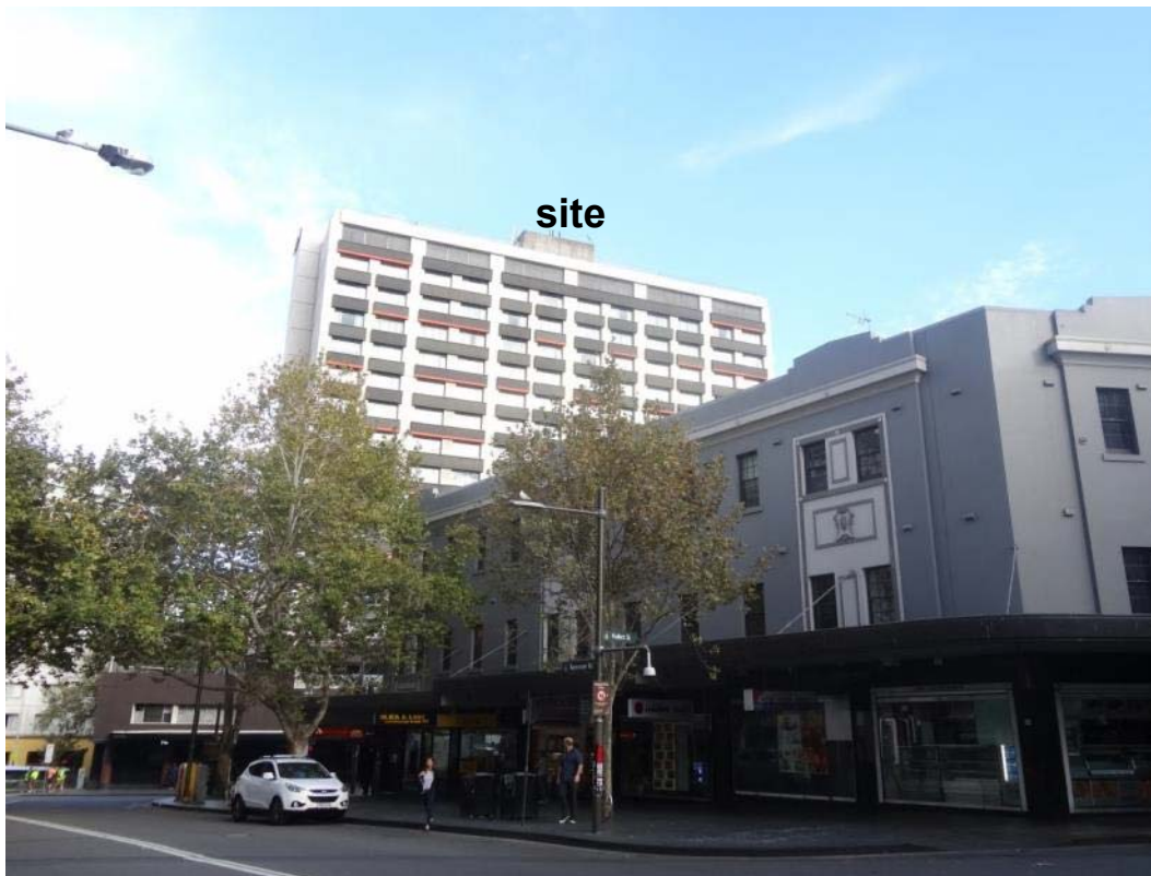
Figure 4: View of the site, looking west from Bayswater Road
