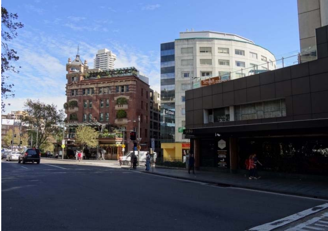
Figure 9: View of the Kings Cross Hotel, a local heritage item located to the south west of the site
