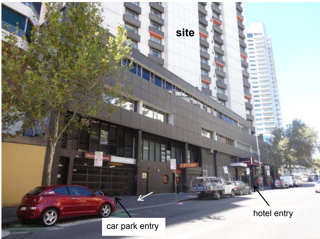
Figure 6: View of Victoria Street west facade showing 3 storey podium with entries
